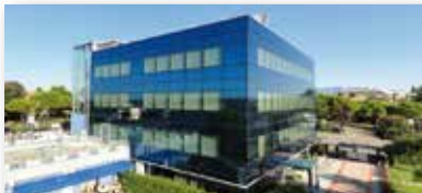
ROVER Laboratories and offices
