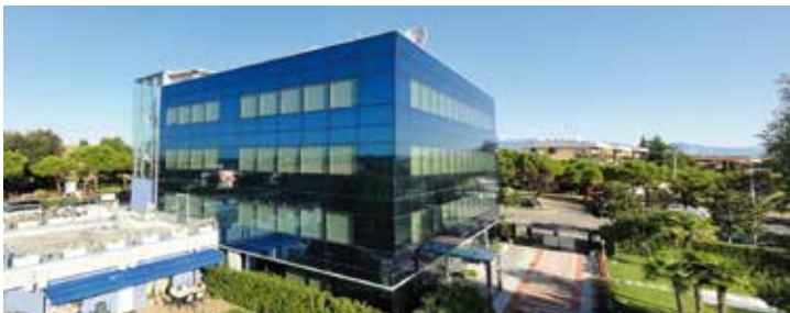
ROVER Laboratories and offices
