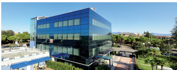
ROVER Laboratories and offices
