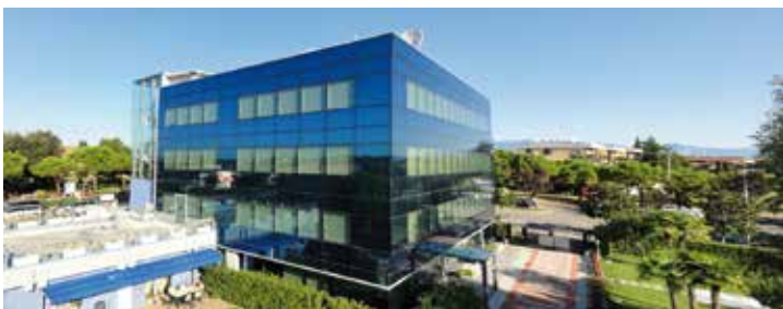
ROVER Laboratories and offices
