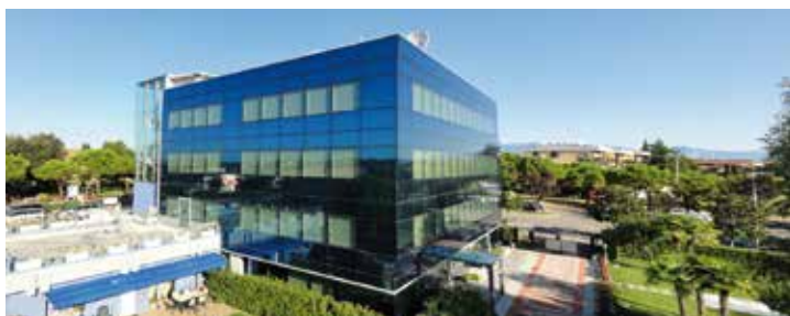
ROVER Laboratories and offices
